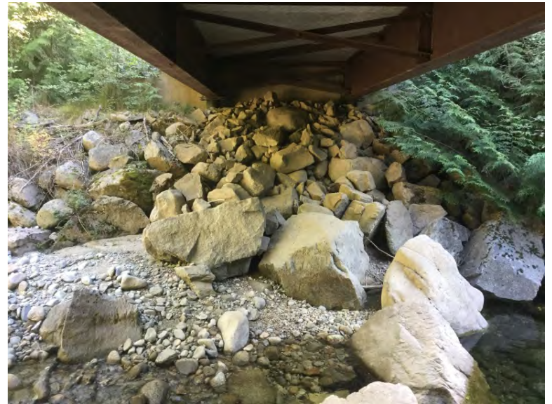
Left Bank Abutment when facing downstream
