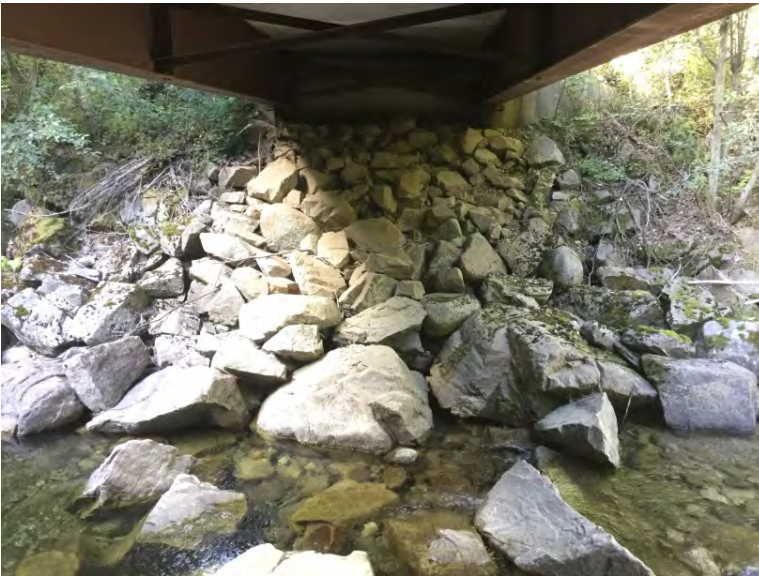
Right Bank Abutment when facing downstream
